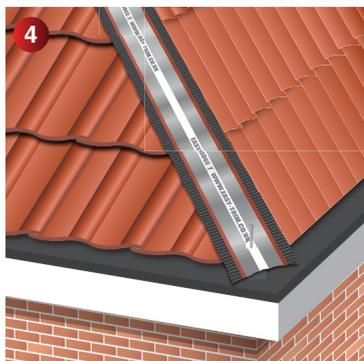
**4** Roll out the Easy-Ridge F roll centrally across the entire length of the ridge batten, using the white spine of the roll as a guide over the ridge batten. Secure the roll by nailing through the white spine using corrosion resistant nails provided. All joints in the ridge roll must be overlapped by 75mm min. Leave a 75mm long strip of the roll at each end of the hip.
